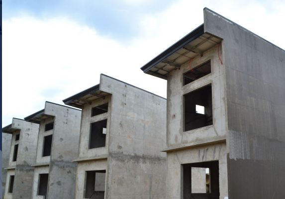
Precast Concrete Construction
